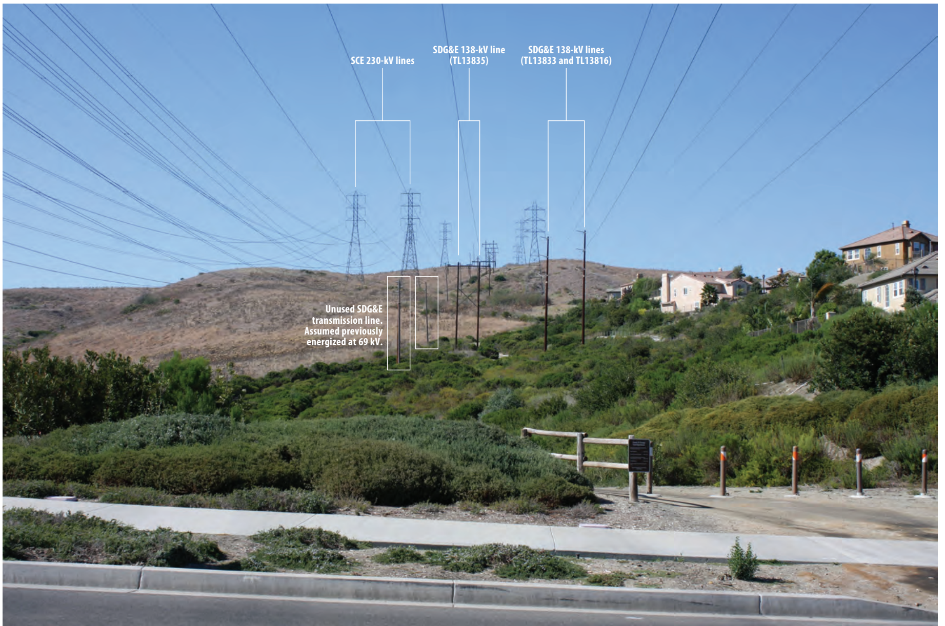
Existing view from Calle Saluda at Prima Desecha Trail looking northwest
